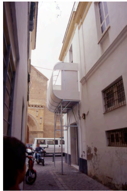
Figure 4: The Scaffolding Housing project
