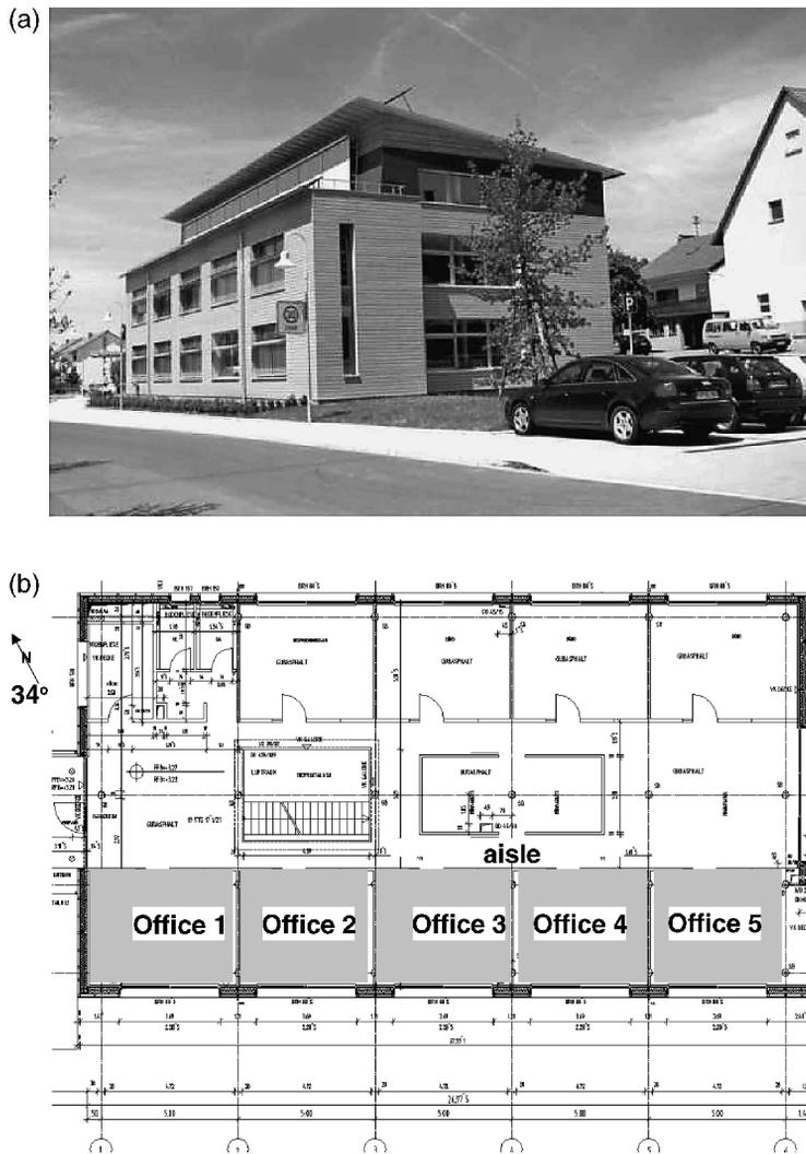
**Figure 4** (a) Photograph of the monitored Lamparter building (architects: Meier-Weinbrenner-Single, Nürtingen, Germany). (b) Typical floor plan of the building. The field study was carried out in the offices with the SSW facade orientation (marked grey). (c) Daylighting concept in the offices. (d) Example video capture from the data acquisition system for the blind settings
