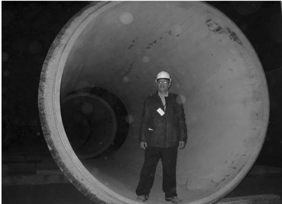
Figure 4.3 Four meter prestressed concrete water pipe used in the great man made river project
