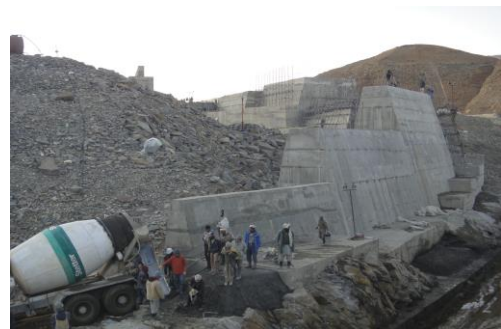
Figure 7. Concreting upstream area
