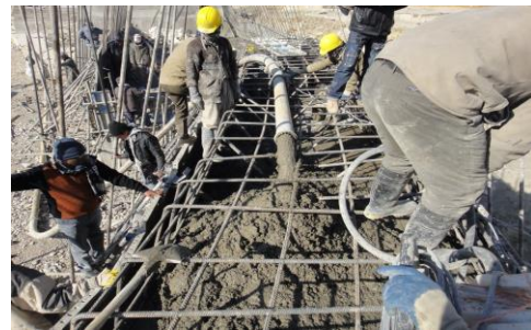
Figure 5. Placement of concrete
