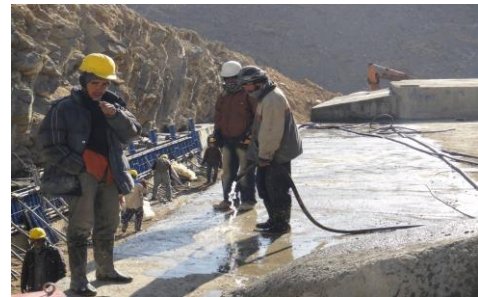
Figure 6. Curing of concrete
