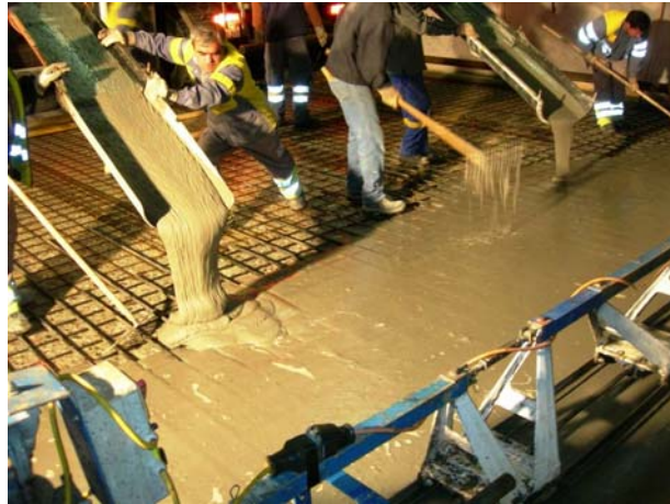
Figure 6: Cross section (dimensions in cm) with UHPFRC layer (in grey) and view of UHPFRC casting performed in autumn 2007.
