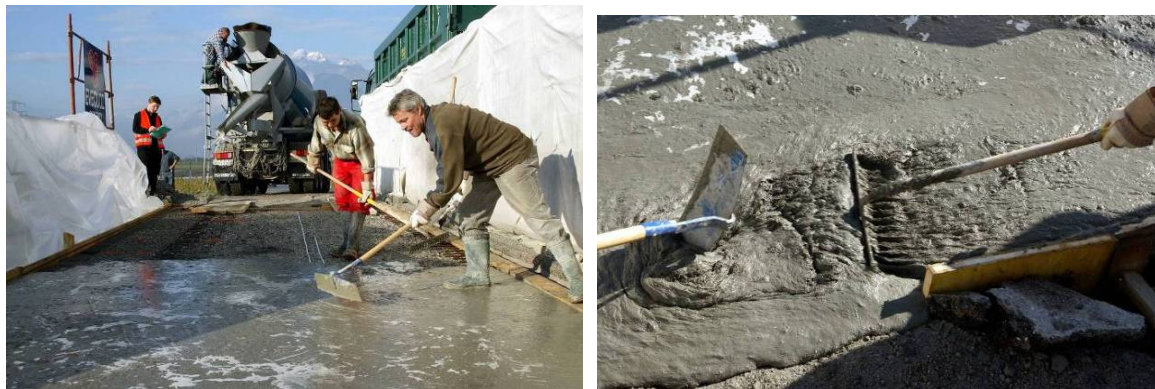
Figure 3: UHPFRC casting and handling of UHPFRC using simple tools.
