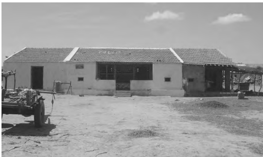
An SHA house in Rapar Taluka (Kachch district)
