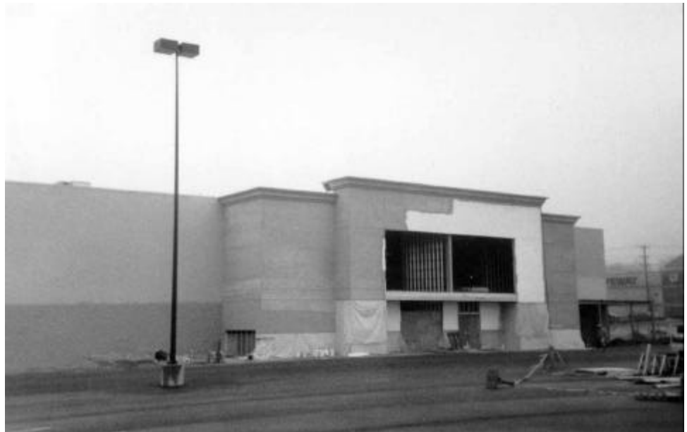
Sam's Club under construction in the redevelopment of Westview Shopping Center along Baltimore National Pike (Route 40 West).
