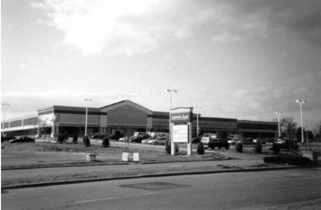
Conversion of a former Hechinger store to a Super Fresh Grocery store. This adaptive reuse project is adjacent to the Security Square Mall in Baltimore County, Maryland.
