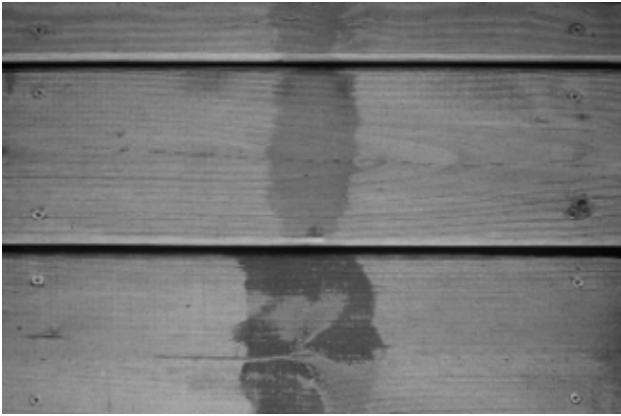
Figure 6—Lap marks on deck finished with a semitransparent stain.
