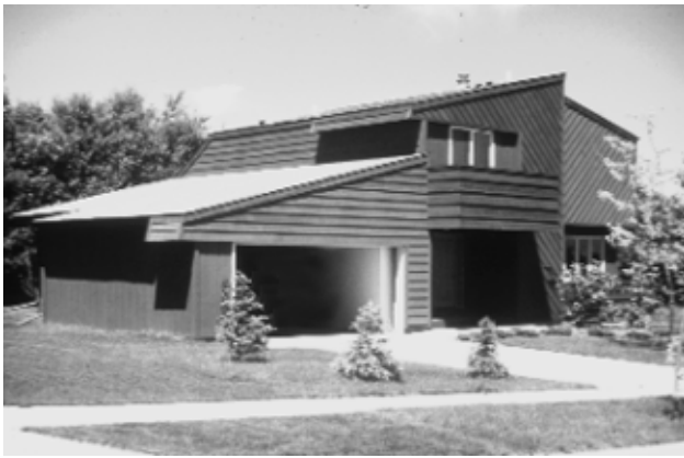
Figure 2—Structure finished with a semitransparent stain.
