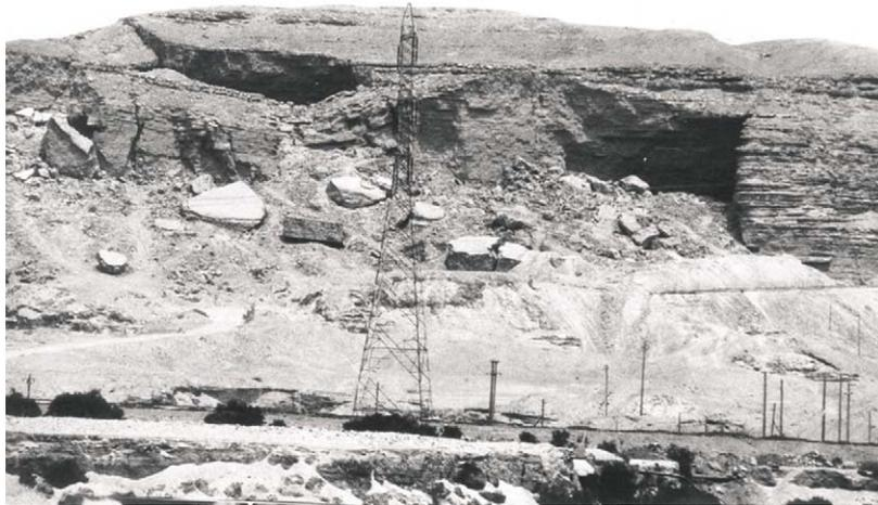
Fig. 9. Partly collapsed large underground quarries within the limestone escarpment of Tura, southeast of Cairo. The gallery quarries continue some 80 m into the escarpment.
