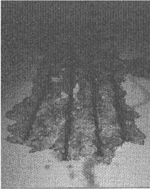
**Photo 1** Corrosion of reinforcing steel
