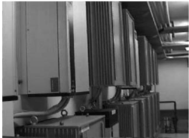
**Figure 3: An array of frequency converters**
