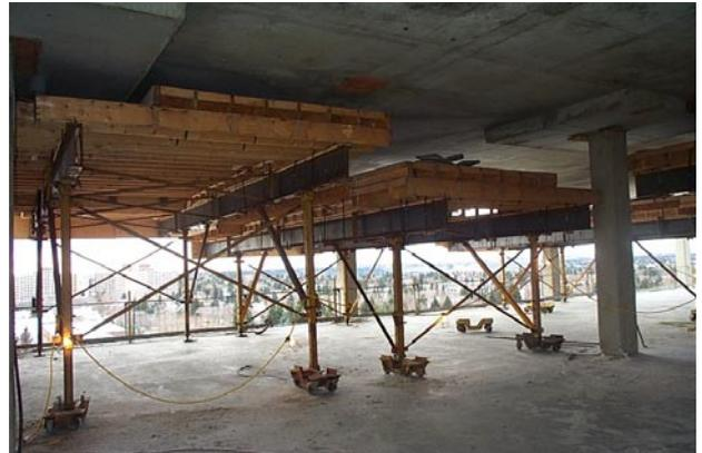
Figure 3: Slab Fly Forms Used For ECERF Building Floor Construction
