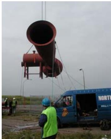
**Illustration 2:** The HydroVenturi alpha test unit being sited in Grimsby, England, comprises a traditional Venturi tube with air storage tank integrated on the left.
