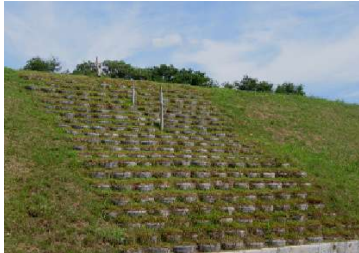
Figure 6: The completed structure
