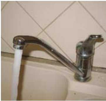
Photo C: Aerator in kitchen tap reduces water use.
