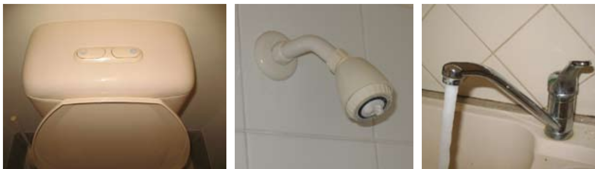
Figure 5.7: Images of a dual flush toilet, water-efficient showerhead and kitchen aerator
