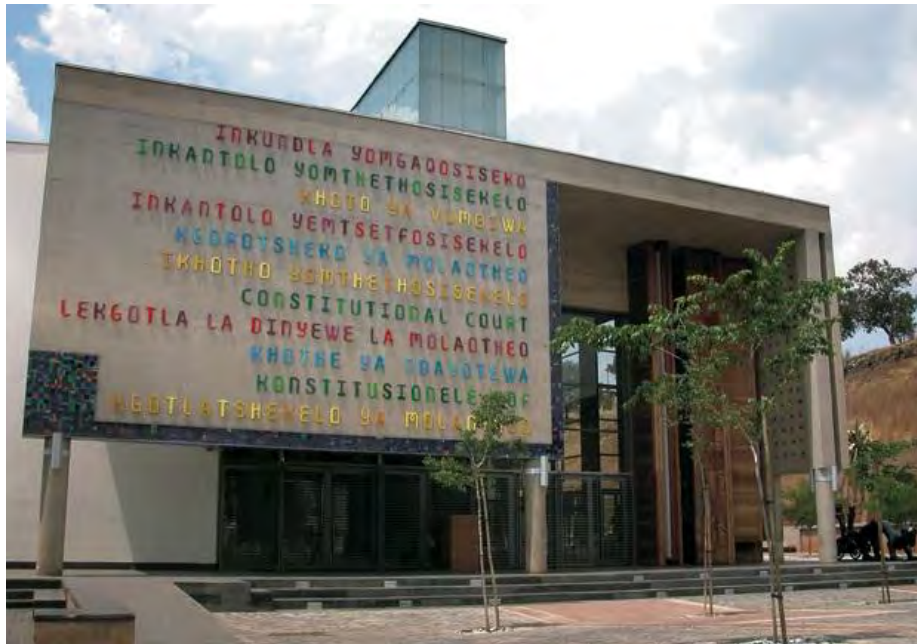
Figure 25: main entrance into the building.
