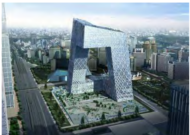
Figure 15: Koolhaus's Television Tower Source: http://crgp.stanford.edu
