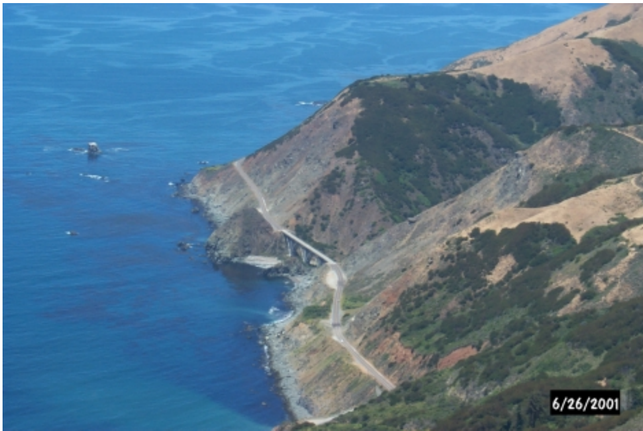
Figure 1. View of Highway 1 at the mouth of Big Creek, where the road crosses several extensive landslide areas south of the bridge and a large area of rock fall and debris slides north of the bridge. View looking Northwest. Photo by C.J. Wills.
