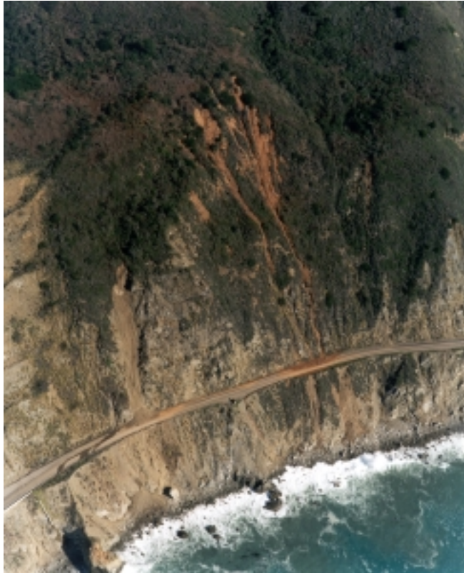
Figure 5. Cut slopes south of Limekiln State Park were subject to small shallow landslides in 1998. These slides included debris slides from loose, slightly weathered rock, on the left, and debris flows from older, dark reddish brown colluvium, on the right. Photo by L. Highland, Caltrans.
