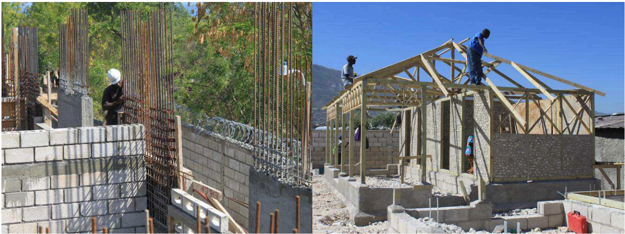
1. Usual reinforced concrete system and CRAterre system
