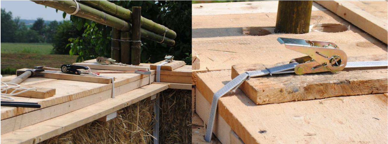
6. Wooden structure at the top of straw bales walls
