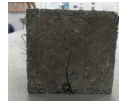
Fig. 7: Macro Fibre concrete after test
