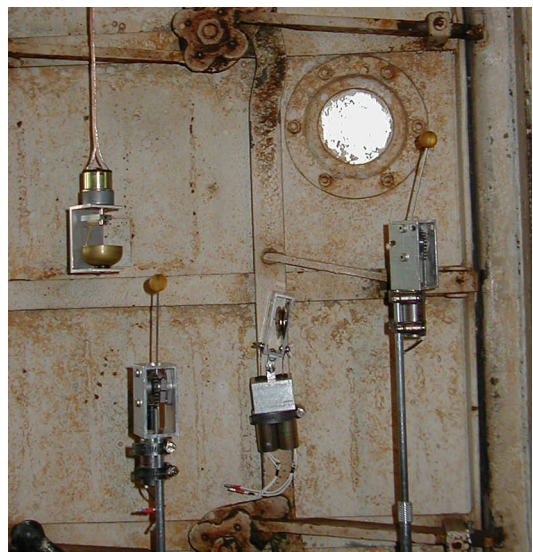
Figure 5: Several ModBots in installation
