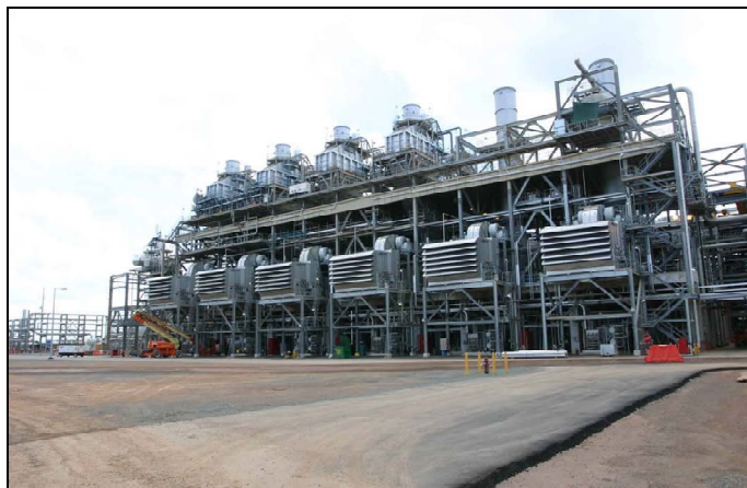
Figure 4. Photograph of compressor trains at Darwin LNG. View of the inlet filter ducts and once through steam generators (heat recovery units) on four gas turbines on the left.
