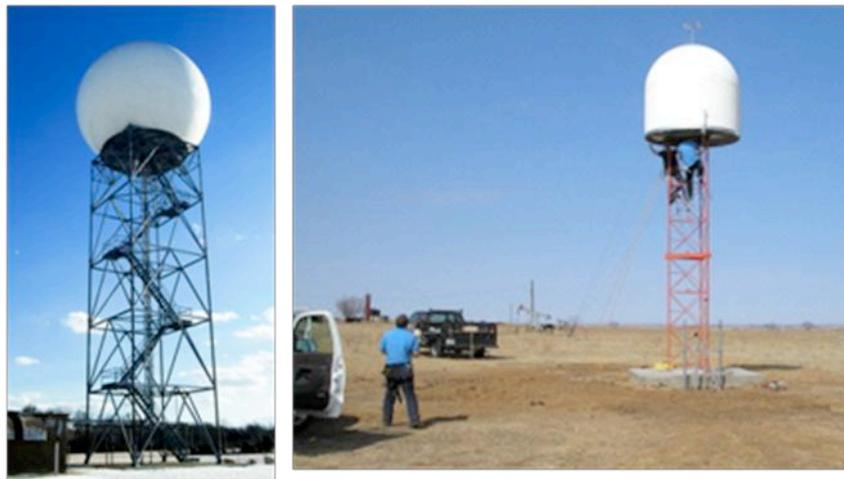
Figure 6.1: The 10 m diameter radome of a long-range S-band WSR-88D/NEXRAD radar is shown at left. A small CASA radar is shown at right atop an 8 m tower.
