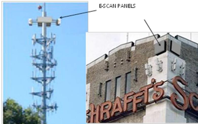
Figure 7.1. Artistic concept of CASA radar panels attached to a cellular telephone tower and the sides of a building.
