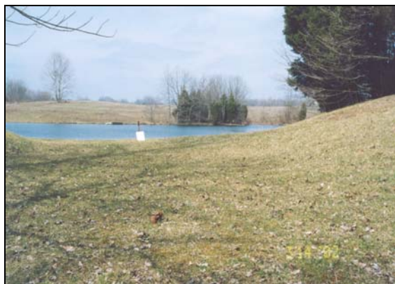
Figure 2-10 Grass-lined emergency spillway.
