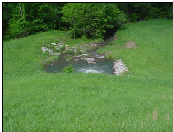
Figure 2-5 Riprap-lined stilling basin at spillway outlet.
