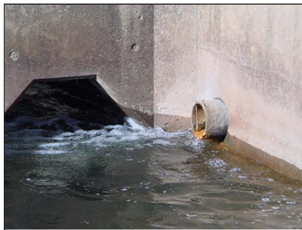
Figure 2-6 Toe drain pipe outlet (right) located near principal spillway outlet.
