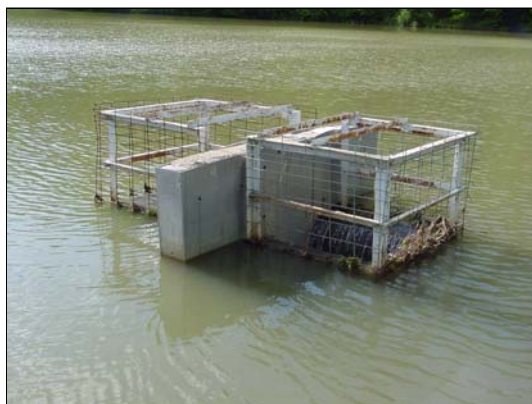
Figure 2-7 Trash racks on riser spillway structure.
