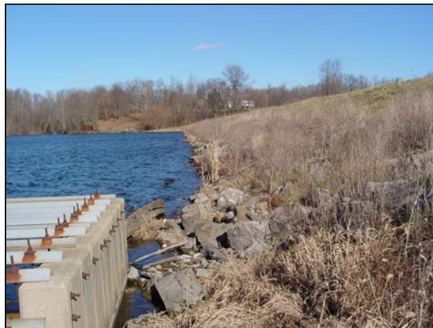
Figure 1-5 Embankment dam with a concrete riser is a common type of dam requiring inspection in Indiana.
