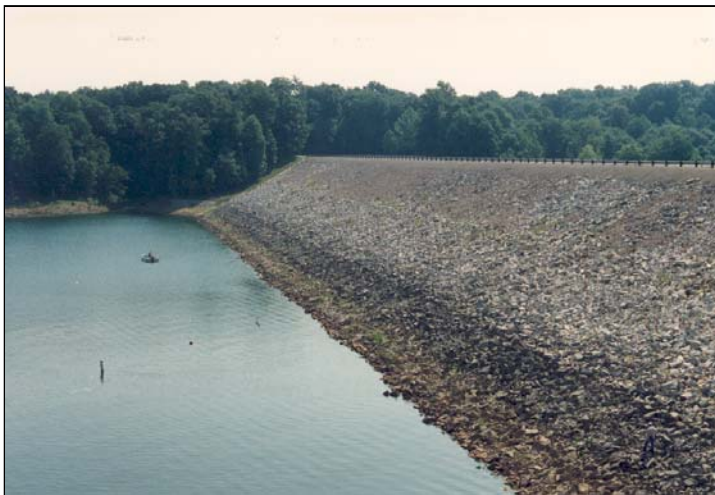
Figure 2-11 Riprap slope protection on an embankment dam.
