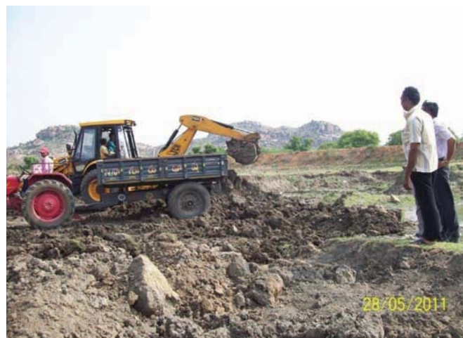
FIGURE B.11: Tank Silt Applied to Enhance Soil Fertility and Increase Water Harvesting Capacity of Tanks in Kadapa, Andhra Pradesh
