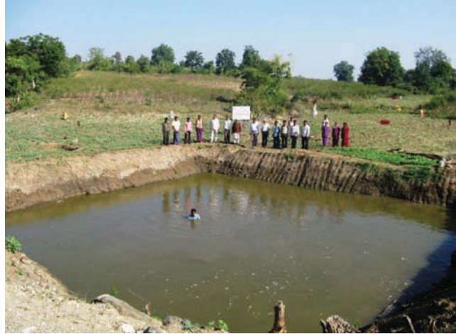
FIGURE B.10: Farm Ponds for Harvesting Runoff and Recycling During Midterm Droughts in Adilabad, Andhra Pradesh, and a Village Pond in Uttarakhand
