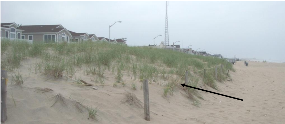
Figure 5.5: Sand fence slats replaced by rope on the seaward side of the dune to control access to the dune (Manasquan, NJ)
