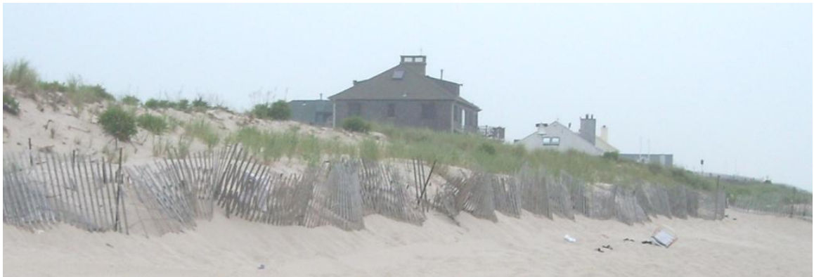
Figure 5.4: Damaged or decaying fences still important in organizing and compartmentalizing space (Brick Township, NJ)
