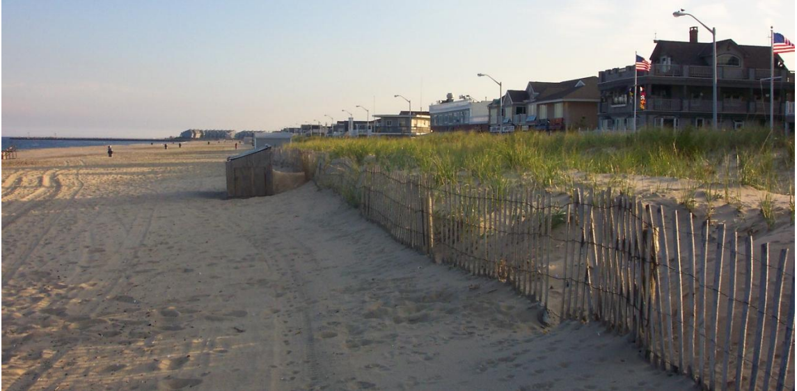
Figure 3.1: Straight wooden slat sand trapping fence at the dune toe. Manasquan, NJ
