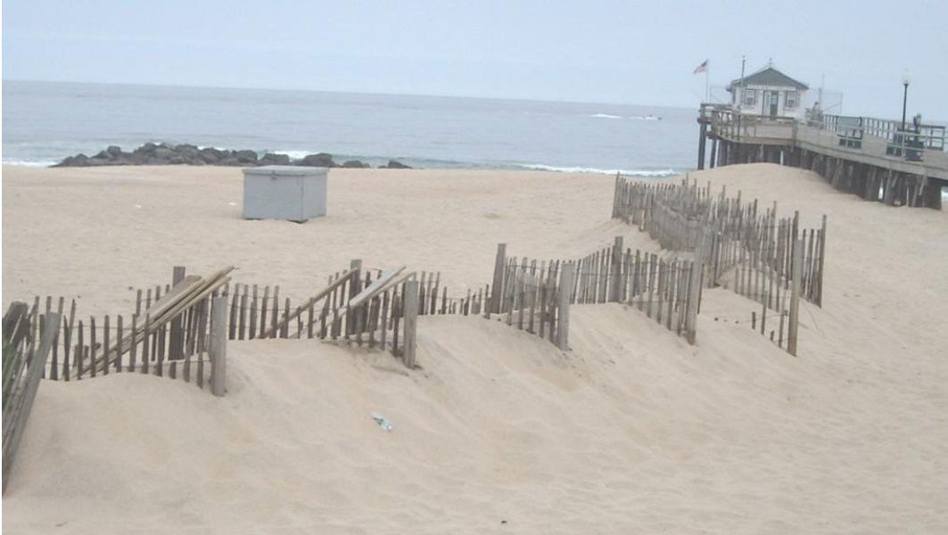
Figure 5.6: Zigzag fences on the middle of the backshore are human intrusions on the beach that form unvegetated dune ridges (Ocean Grove, NJ)
