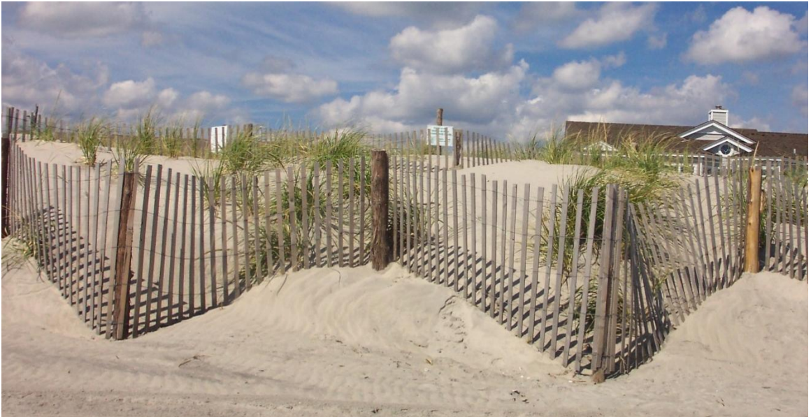
Figure 3.2: Zig-zag fence at the dune toe/foreslope and remnant fence at the dune crest. Stone Harbor, NJ.
