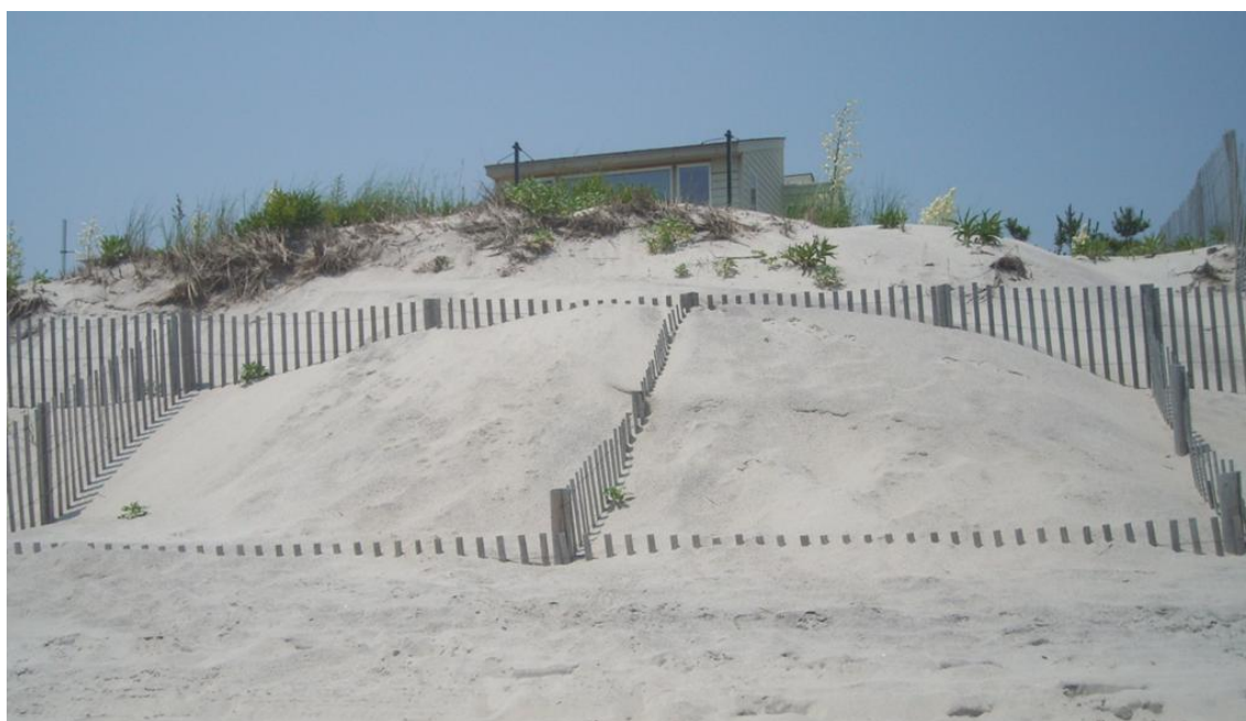
Figure 5.3: Fence configuration observed in 2008 field reconnaissance but not in 2002 video inventory, double line of shore-parallel straight fences partitioned into rectangular compartments (Loveladies Beach, Long Beach Township, NJ)
