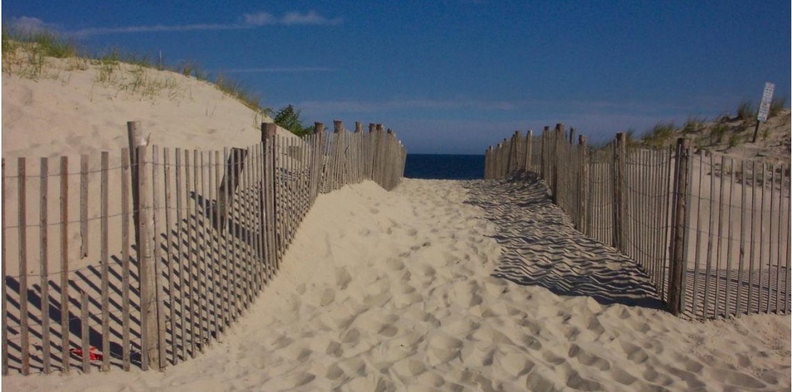
Figure 3.5: Walkway fence arrangement perpendicular to the shore, NJ.
