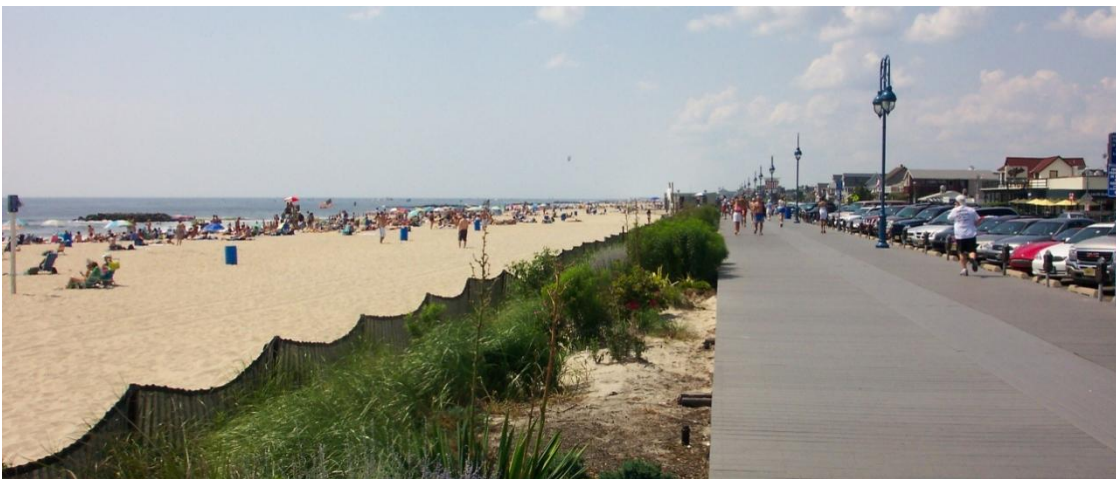
Figure 3.6: Fence placed to prevent sand inundation and control pedestrian access to the beach through boardwalk, Belmar, NJ.
