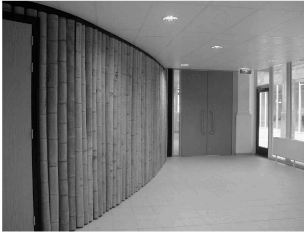
Figure 9. Bamboo culm as a finishing material (photo by Hulshof architects).
