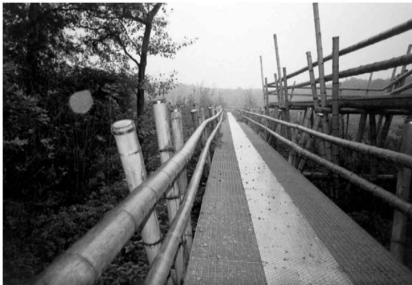
Figure 1. Bamboo bridge in the Amsterdamse Bos (photo by Pablo van der Lugt).
