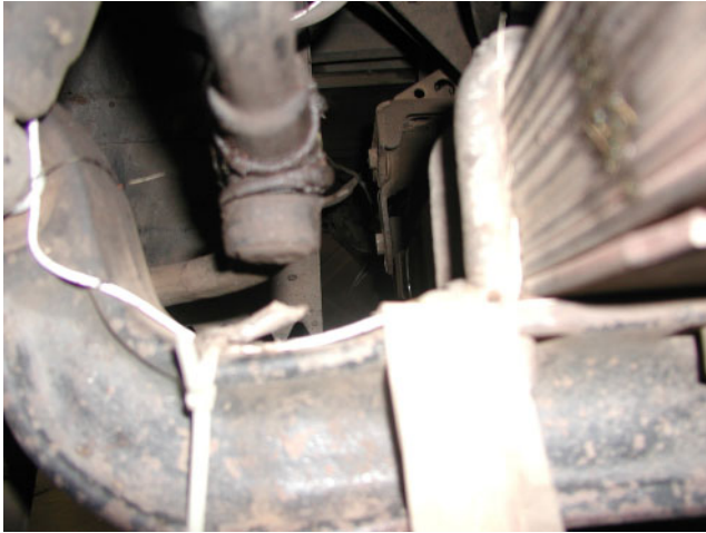
Fig. 2 Accelerometer location on the front axle
