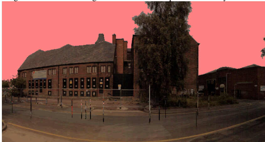
Figure 5 The back side of the Jactin House building in Manchester
