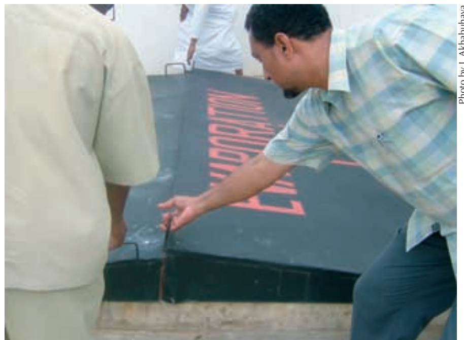
Evaporation basin – disposal facility: this is one of the techniques for safe disposal of plant effluents.
