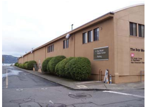
Northwest elevation, looking east, 100_1414
