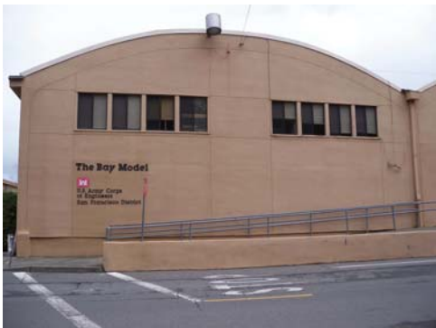
Detail of southwest elevation, 100_1413
