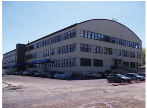
Northeast and northwest elevations, 100_2576
