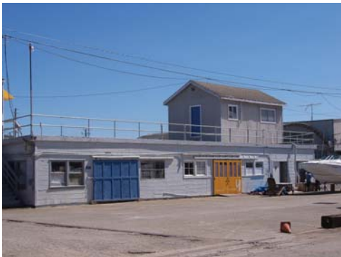
Shipway Bldg. No. 1, 100_2537
