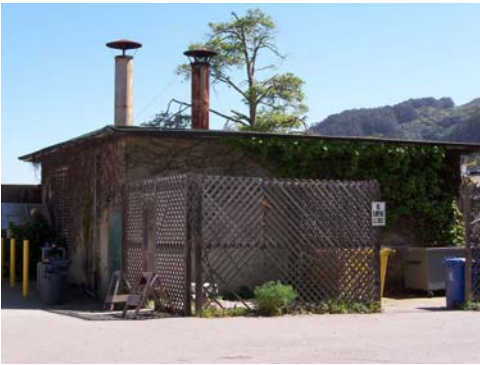
Incinerator at rear, 100_2636
