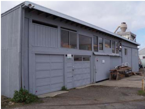
Oil storage building, 100_1564
