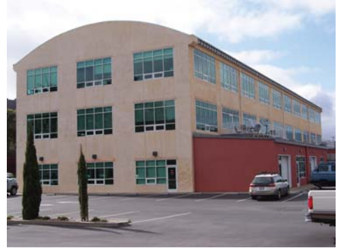
North and west elevations, 100_1555
