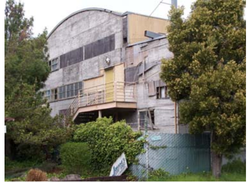
Portion of southwest elevation, 100_1527
