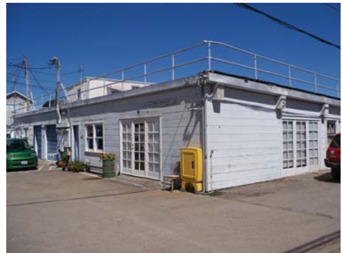
Shipway Bldg. No. 2, 100_2543
