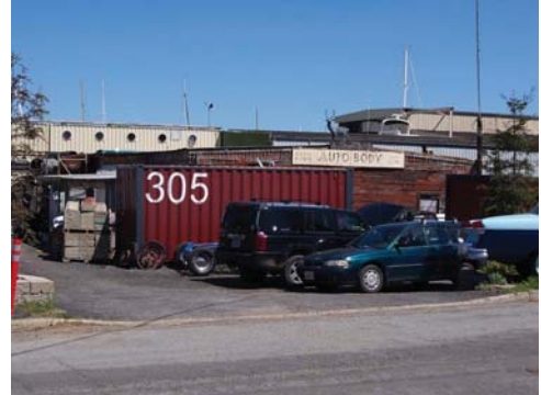
Southwest elevation and part of northwest elevation 100_2599
