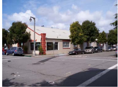
Southeast elevation, looking east, 100_1911
