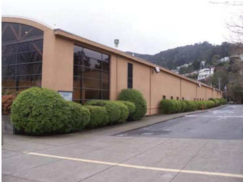
Northwest elevation looking west, 100_1418
