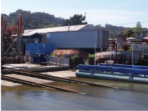
Way No.3, looking northwest, 100_2669
