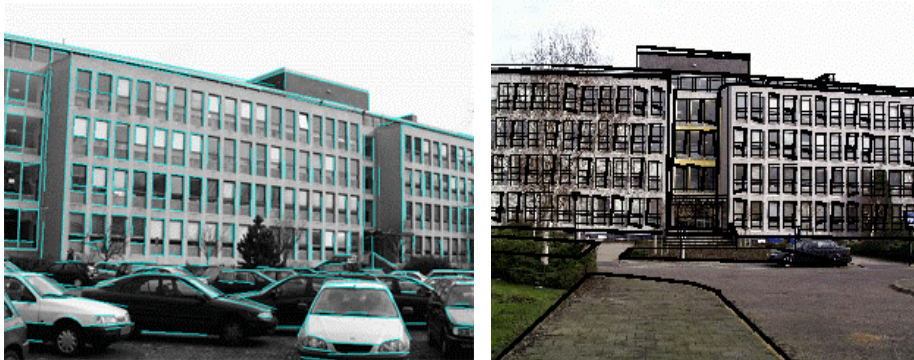
Figure 3. Lines extracted from the camera images (left) and from the GIS database (right). Matching those lines gives an accurate estimation of the camera position and orientation.
