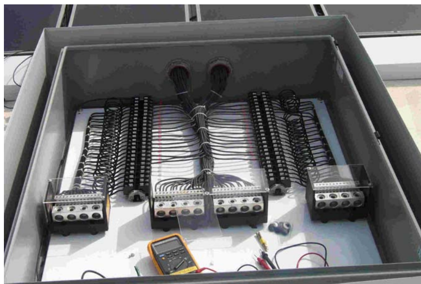
Fig. 16: Photo of a wiring ‘combiner box’ housing the terminations for 17 high-voltage module-strings in a large array. In this case, each module string had twelve 150- W_p crystalline silicon modules connected in series.
