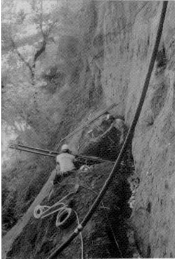
Figure 3 Tieback drilling rig, waterjet assist.
