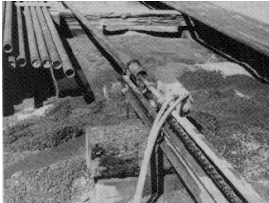
Figure 1. Cleaning cement filled pipe with high velocity waterjets in Phase 1.
