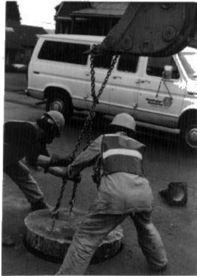
Figure 4. Pavement Plug Removal
