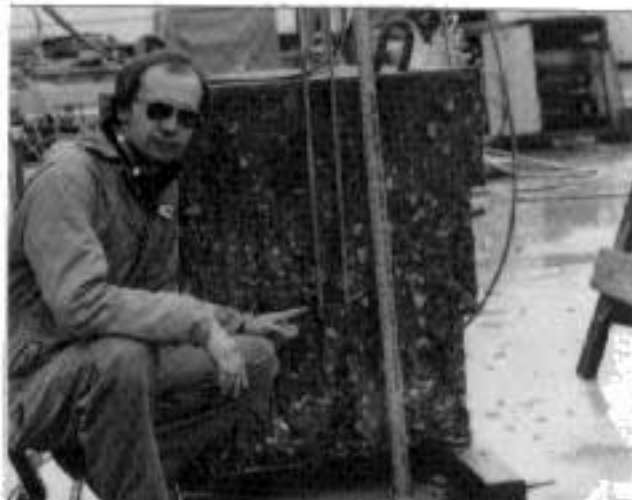
c. Nozzles next to the cut face
