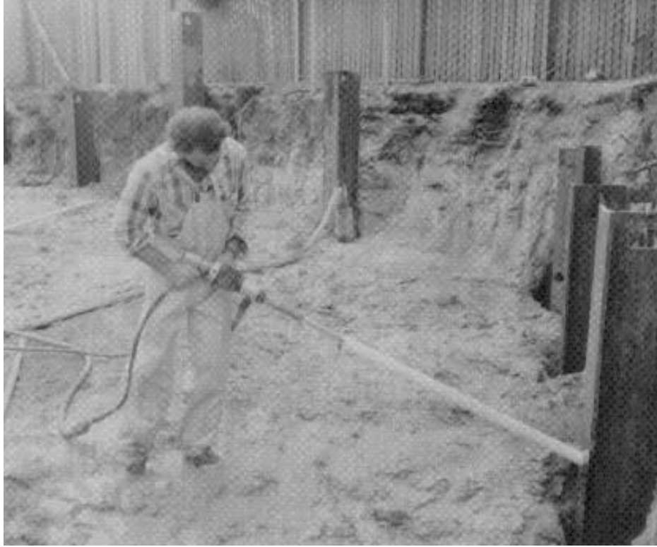
Figure 1 Handheld waterjet assisted drilling of tieback anchors.
