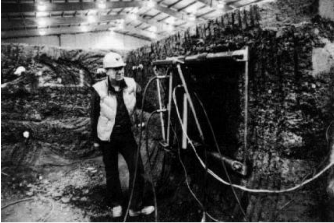
Figure 2. Portable in-seam tester mounted on coalcrete block.
