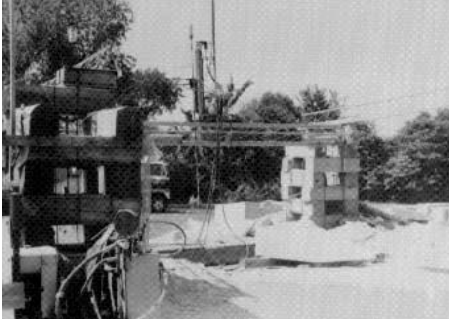
Figure 4. General area of cutting rig.
