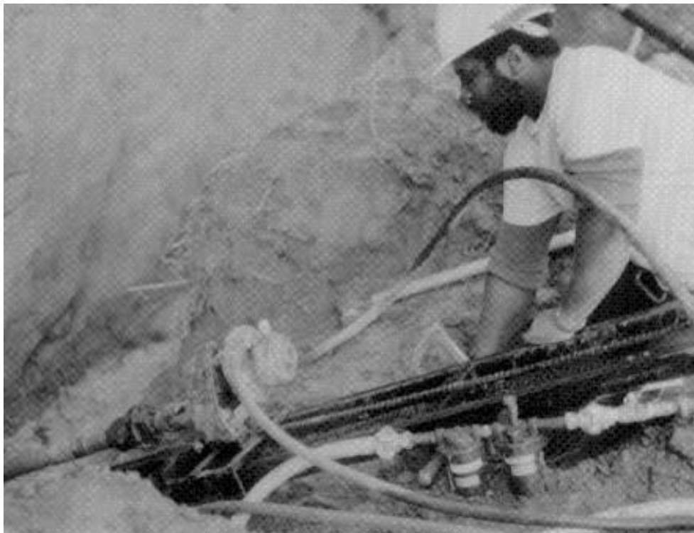
Figure 2 Waterjet assisted drill rig, hand fed.
