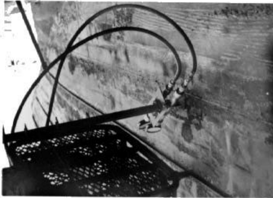
Figure 3 - SERVOJET Array Shown Mounted on Basket of "High Reach" Machine
