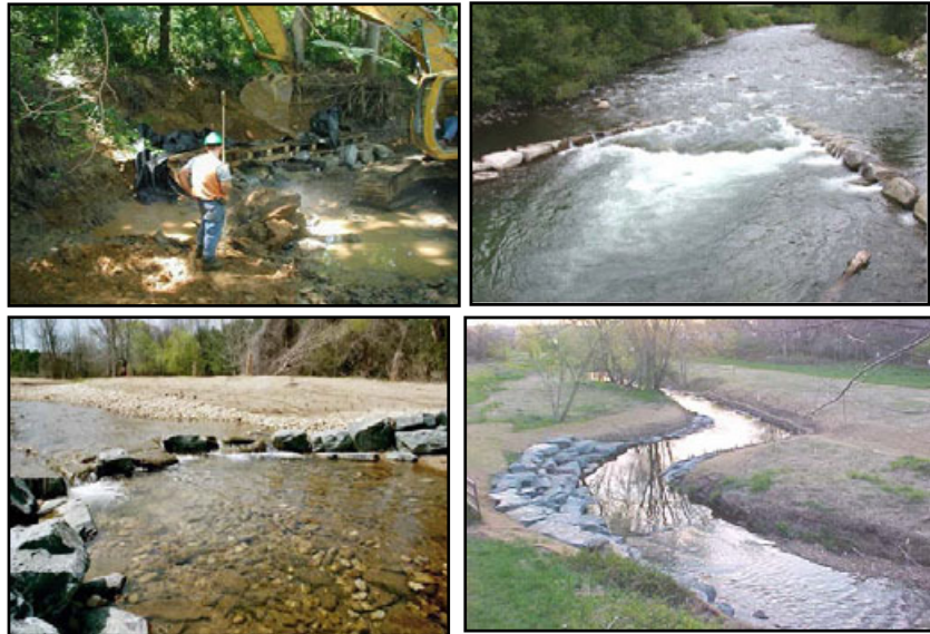
Fig. 2 Photographs of restoration projects in progress or completed to enhance habitat heterogeneity. Upper left: large equipment is typically used to re-configure and create artificial pools and habitat structures such as the wooden framework that will be used to create under-bank openings for biota. Upper right: rock weirs placed in the channel to deflect flows and add variable flow habitats. Lower right: artificial meanders created by re-configuring the channel. Lower left: in-stream rock structures to create shallow pools downstream.
