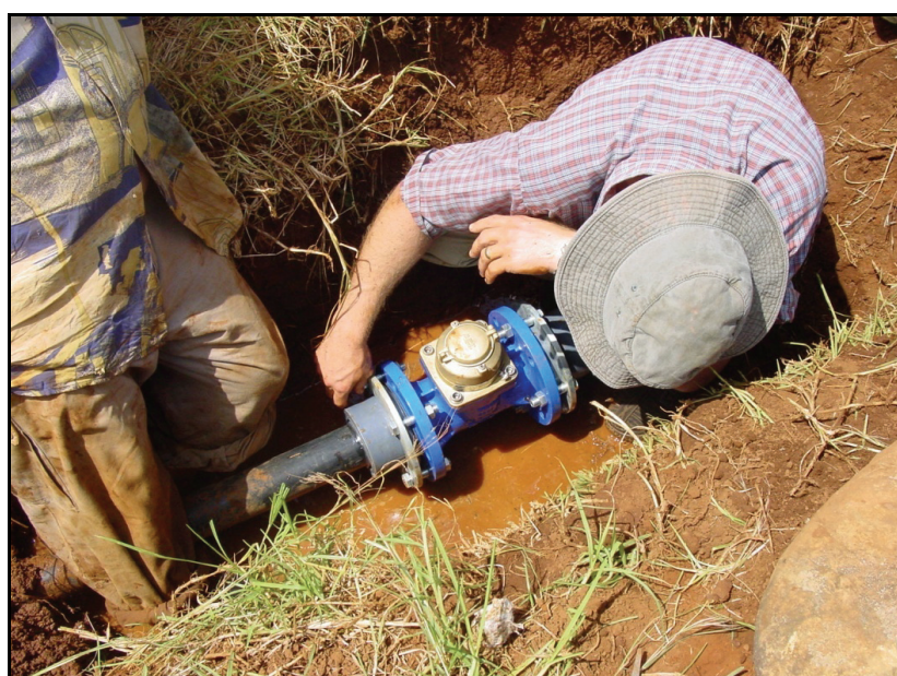
Figure 4.7 The installation of the flow meter at Ntembeni community gardens
