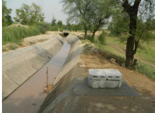
Fig. 11: Photograph of 5R distributary and stilling well.
