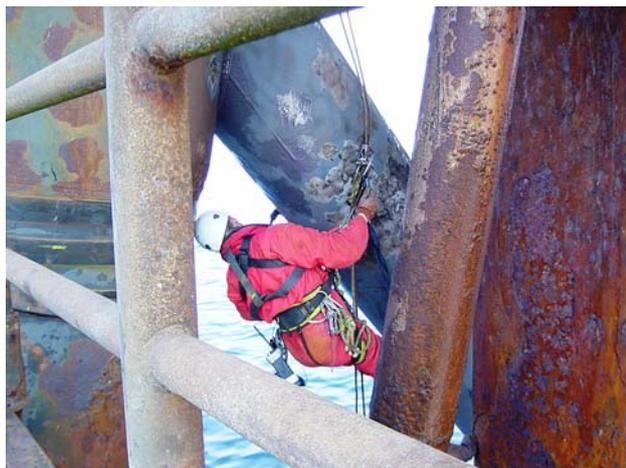
**Fig. 1: Corrosion of steel on offshore structure due to premature failure of coating. Courtesy of Hempel A/S**
