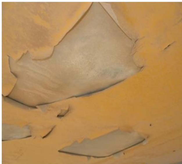
**Fig. 20: Peeling of coating due to inadequate curing conditions**
