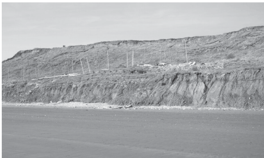
Figure 7. CPK test area photographed during Epoch 2 survey, showing ongoing erosion.
