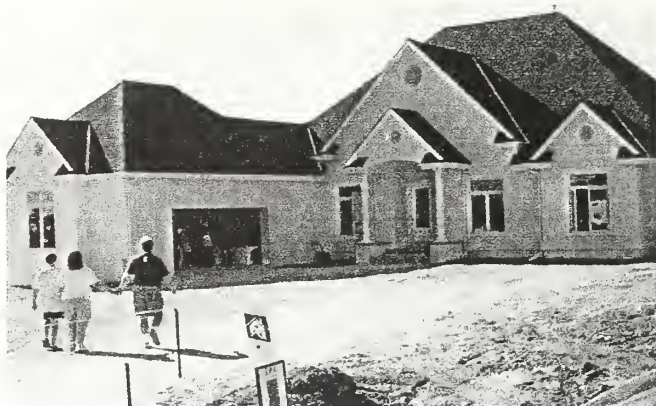
Figure 1-1. New ICF Home in Wisconsin [icfweb.com, 2000]
