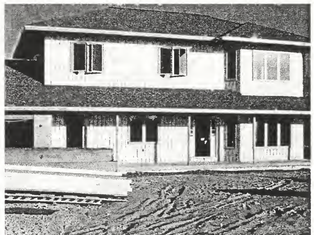
Figure 1-4. New 2-Story ICF Home in Wisconsin [icfweb.com, 2000]
