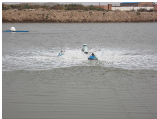
Figure 5. Dissolved oxygen aerator pump working at Tangu fish pond
