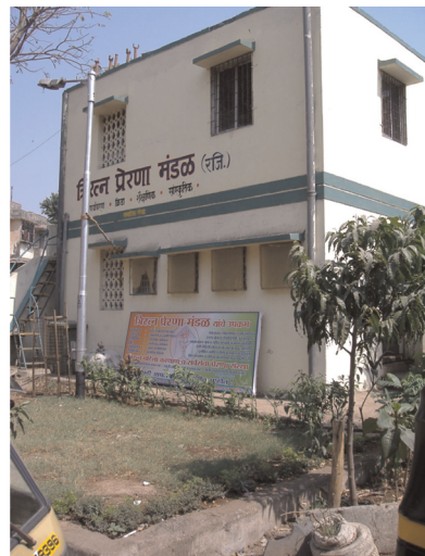
Figure 1. The Triratana Prerana Mandal toilet block, Khotwadi, Mumbai. Photo: author.
