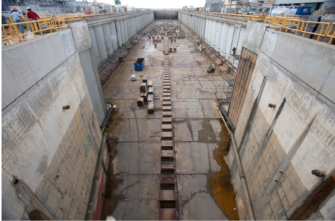
Figure 2: Newport News Shipbuilding Dry Dock #11
