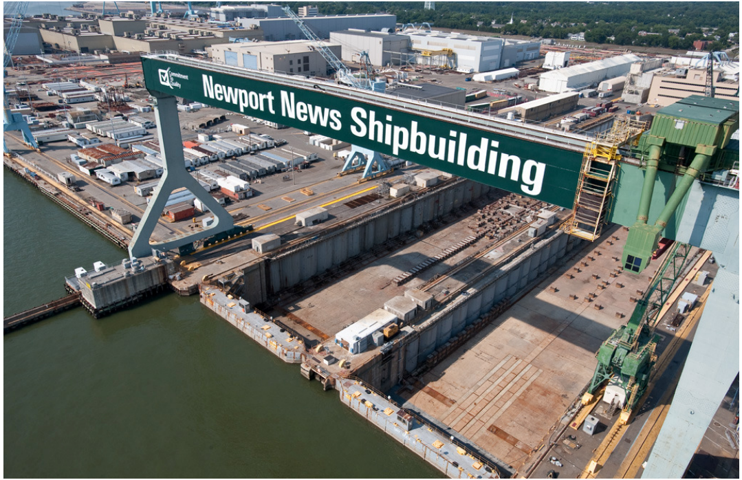
Figure 1: The gantry crane today.
