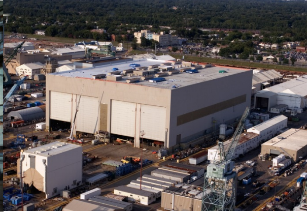
Figure 5: A view of the Module Outfitting Facility
