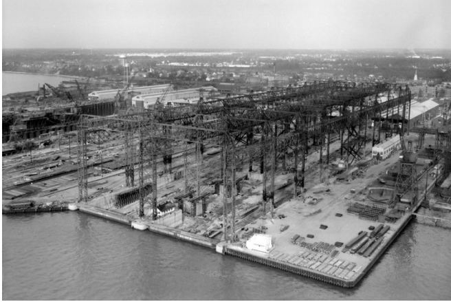
Figure 6: Shipways 8 and 9, along with the trestle above.
