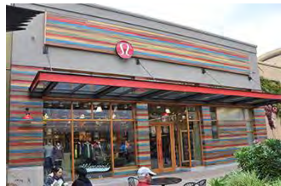
Figure 12. Lululemon store front Lynnwood, Washington – World Mix multi-colored tinted siding. Source: © TerraMai.
