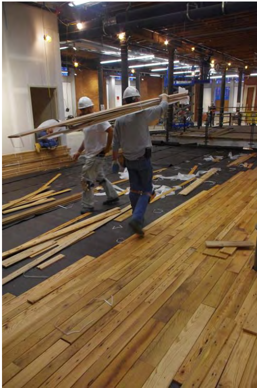
Figure 6. REI SoHo - New York City : Reclaimed wood floor installation. Source: © TerraMai.
