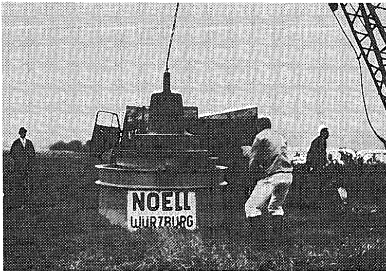
FIG. 1. Driving the steel cylinder into the ground.
