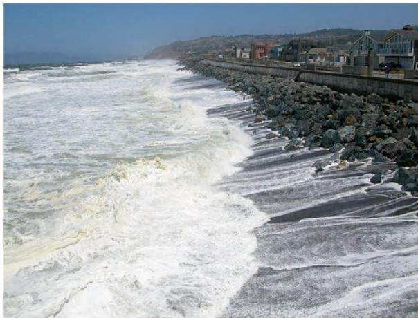
**Figure 10** Beach loss seaward of coastal armoring that includes a seawall and revetment on exposed coast in Pacifica, California, USA. Note the lack of dry sand zones and lateral access for beachgoers.
