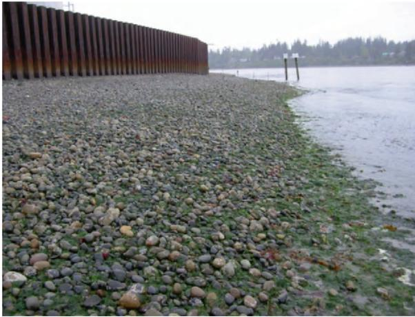
**Figure 4** An intertidal bulkhead constructed of metal sheet pilings located on Puget Sound, Washington, USA. This bulkhead was built to retain contaminated sediments and reduce exchange with the sound.
