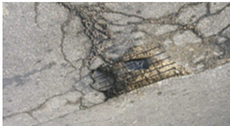
Fig. 10. TSN installed in pothole (road testbed).
