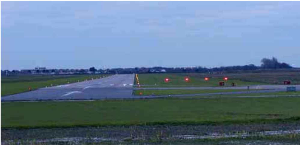
Figure 2a: Photograph of PAPI lights viewed from ground level. Photograph taken at Sussex Flight Centre, Shoreham Airport (December 2006).
