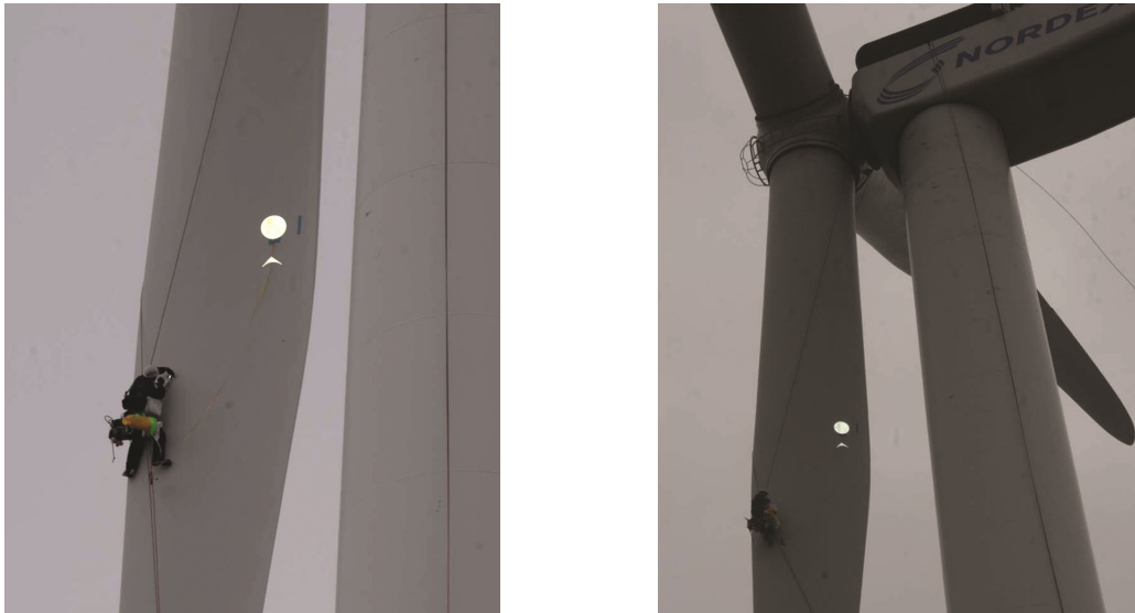
Figure 2.3 a-b. Installation of markers on the wind turbine
