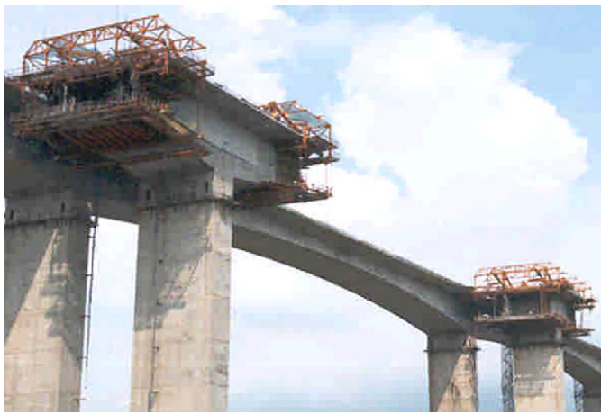
Fig. 5. Balanced Cantilever Method.
