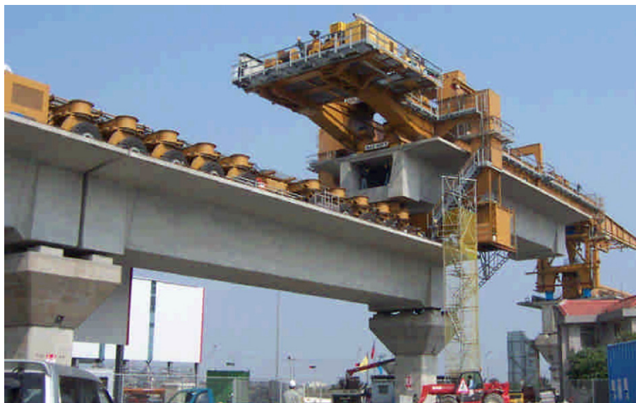
Fig. 3. Full-span and Pre-cast Launching Method.
