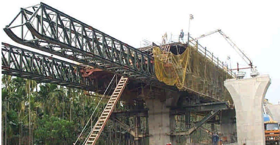
Fig. 4. Advancing Shoring Method.
