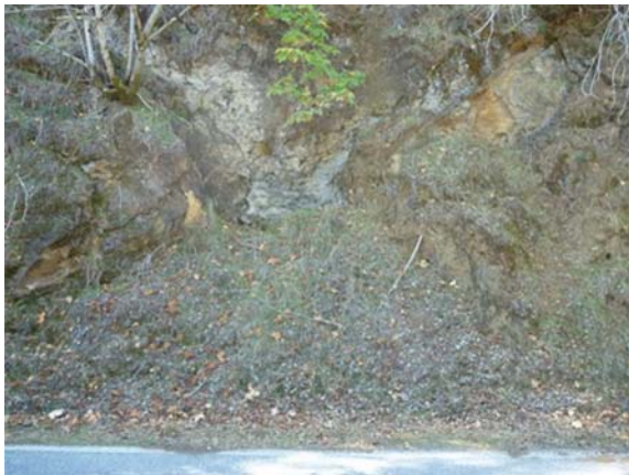
Photo 8: Sealed adit at Road Tunnel
