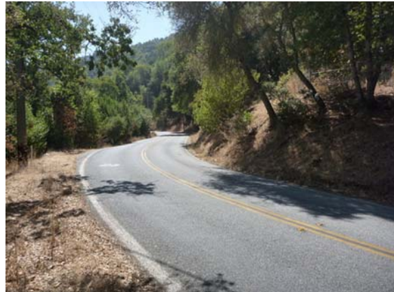
Photo 5: Eastern end of upper embankment below Engine Shaft site to right, and top of lower embankment to left.
