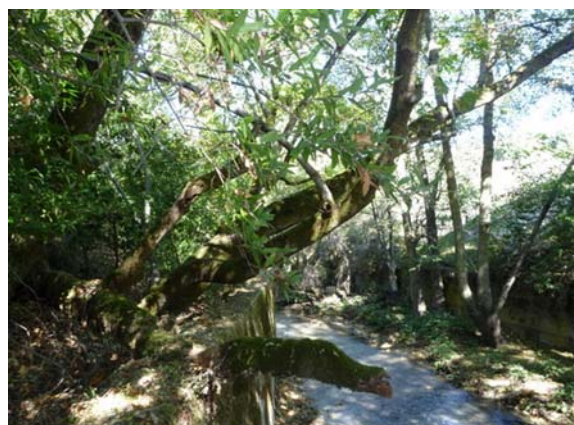
Photo 7: Concrete flume below Hicks Road, lower retained embankment.
